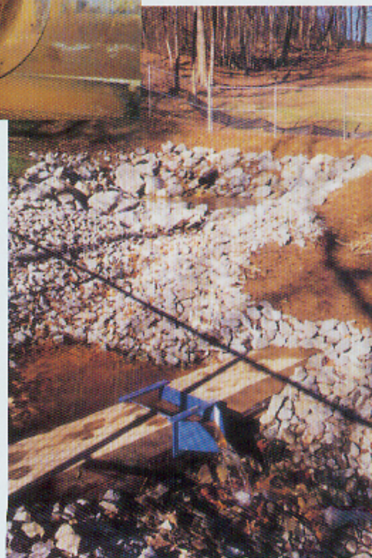
Allegheny Power's Springdale wetland is cost-effectively transforming a metal-bearing leachate (left) into a compliance-quality discharge (below).
