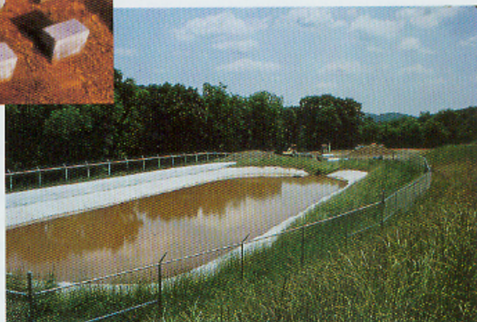
At the Springdale wetland, the leachate is pumped over a concrete aerator on its way to an equalization basin, where most of the iron removal occurs. The aerator introduces the oxygen necessary for the chemical reaction for iron removal.
