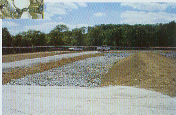
Two rock drains at the Springdale wetland harbor microorganisms that promote manganese removal. Because iron is known to impede manganese uptake and sequestration, the system was designed to remove all iron from the leachate before it enters these drains.
