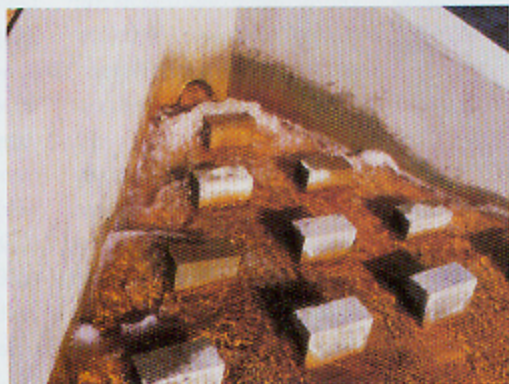
At the Springdale wetland, the leachate is pumped over a concrete aerator on its way to an equalization basin, where most of the iron removal occurs. The aerator introduces the oxygen necessary for the chemical reaction for iron removal.
