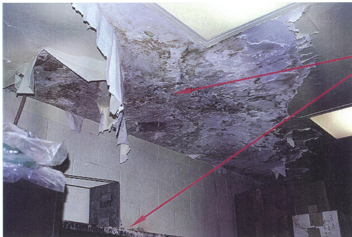
Water Damage to Finishes, Equipment and Furniture
