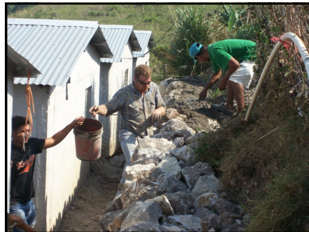
Students work on retaining wall in Honduras
